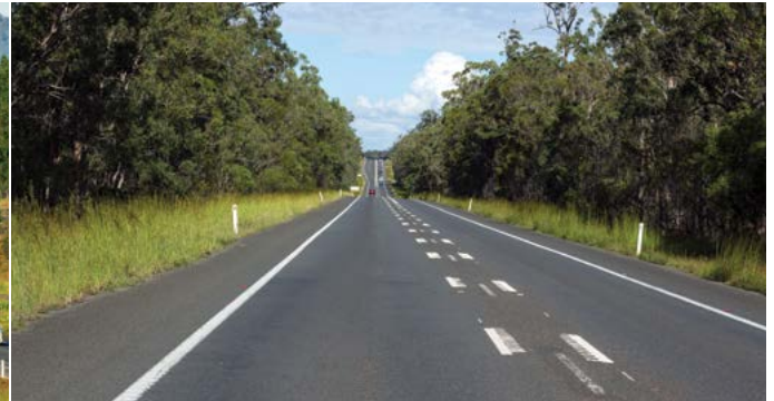
This photo shows a road which has been treated with audible edge and centrelines, and a widened median.
