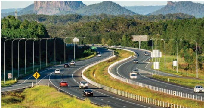
This photo shows a highway treated with flexible wire rope barriers.
