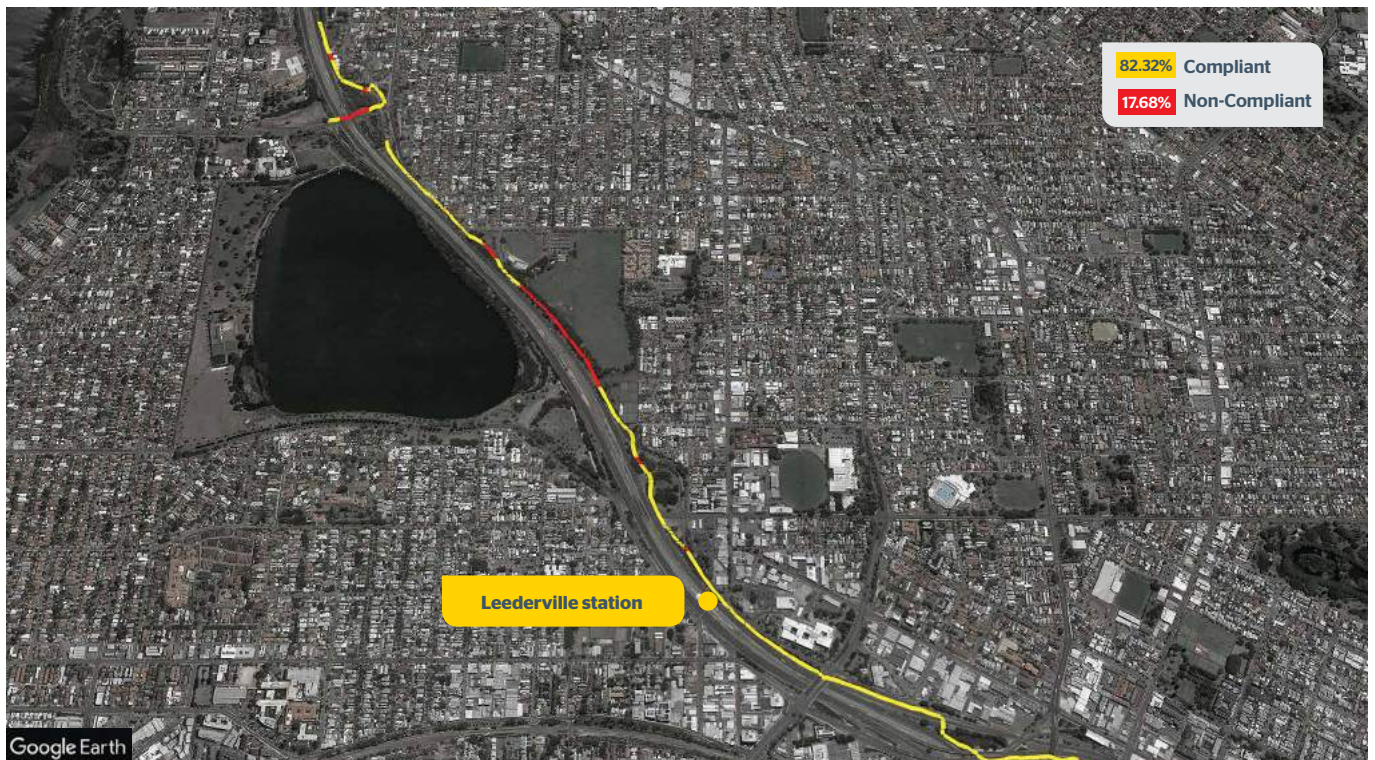
Figure 7 » Mitchell Freeway PSP: Aberdeen Street to Goody Close
